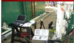
Cable testing using VLF waveform is an accepted and standardized technique. many standard refer to this technique of testing with published methods and parameter to use. . Cable diagnostic testing is possible using VLF test sets where an indicator of overall health of the cable is now possible, cables can be easily and
